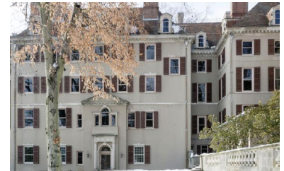
Two windows flanking Winterthur's Port Royal Entrance on the ground level illustrate how the new Plexiglas storm windows will look. Courtesy of Winterthur, photo by Jim Schneck.
